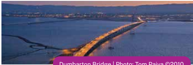
Dumbarton Bridge | Photo: Tom Paiva ©2010
